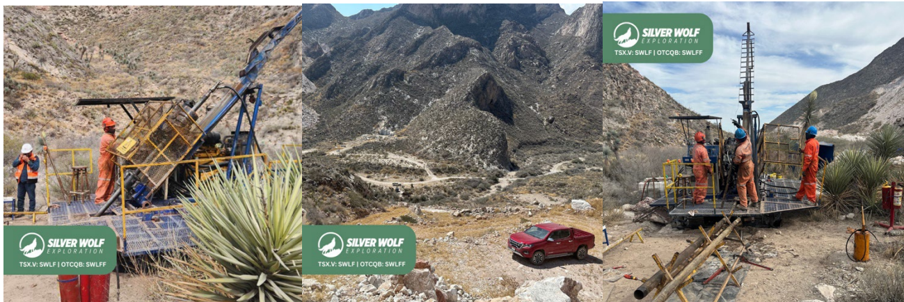
Figure 3: Drilling crews advancing the La Recompensa drill program.
